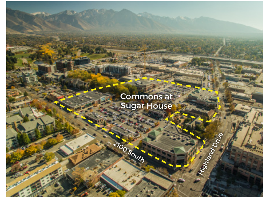
View from directly above the site looking Southeast toward Millcreek.
